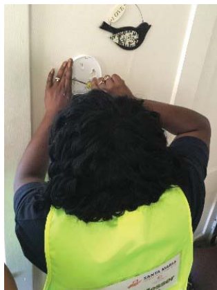
Home Safety Day volunteers helped with installing safety equipment in community homes
